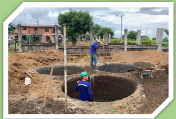
Work begins on Phase 1 of the new vocational education building.
